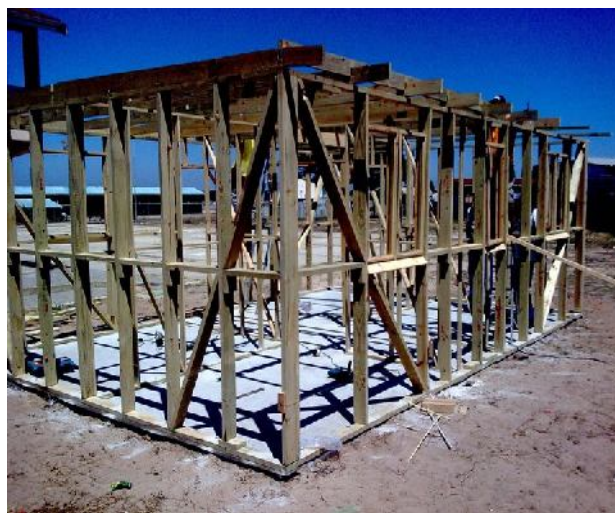
The framework almost completed at Atlantis
